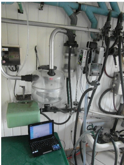
Fig. 1. Programming the quarter pulsator before milking cows (source: author's own photograph)
