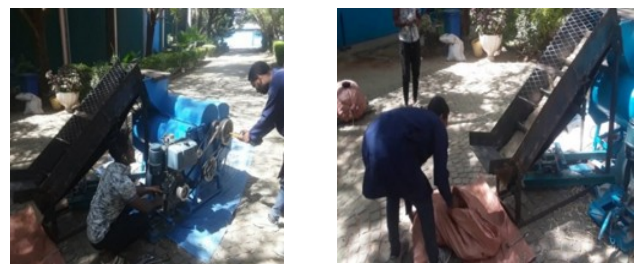
Fig. 12. Picture taken during the performance evaluation on field (source: author's own photographs)
